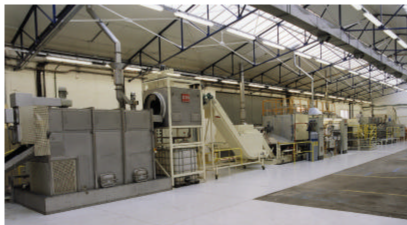
Automatic heat treatment line
